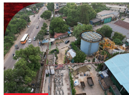
Ariel view of Anaerobic Digester
